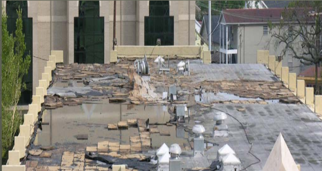
St. Joseph's Roof August 30, 2005
